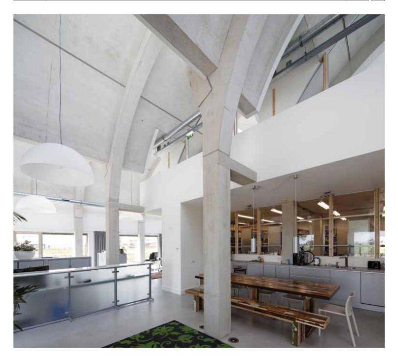
straight parts of the roof are glazed and north facing, allowing daylight into the building while preventing direct sunlight, eliminating the possibility of overheating."
